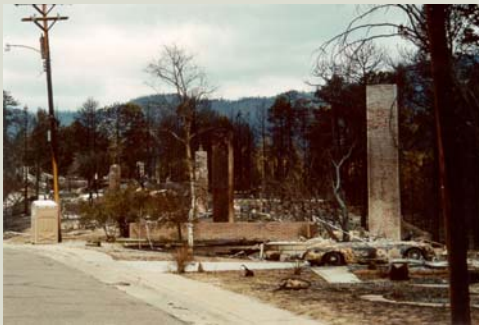
Figure 9. A structure destroyed during the Cerro Grande fire.
