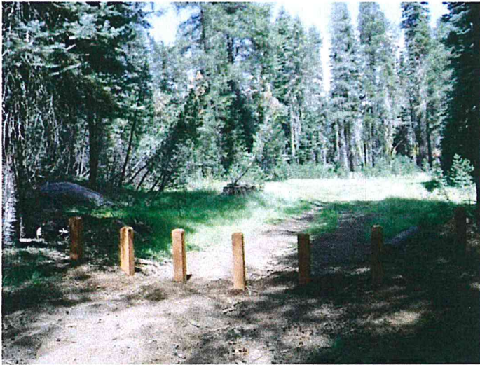
Barrier installation to maintain OHV trail and limit access and protection of meadows. Photo by US Forest Service
